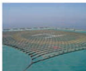
Safety Net of Helicopter Platform.
